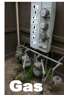
Diagram 2 Gas and Electric Meters
